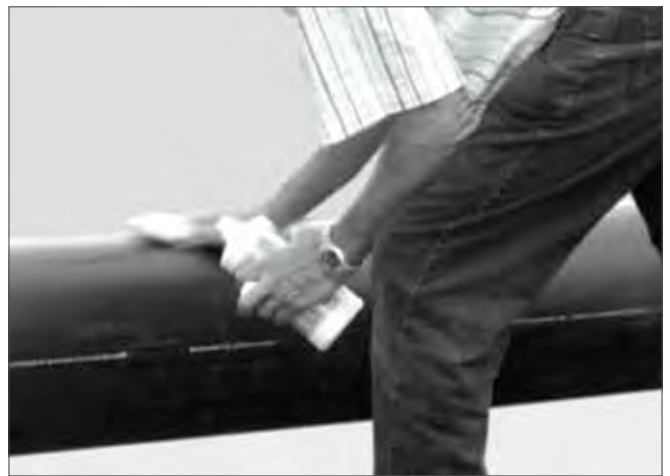
Figure 48: Illustration of Prescribed Cleaning of Pipe Fusion Zone
