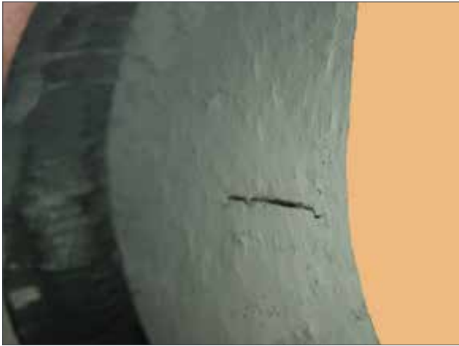
Figure 26: Pipe Failed in Brittle Mode
