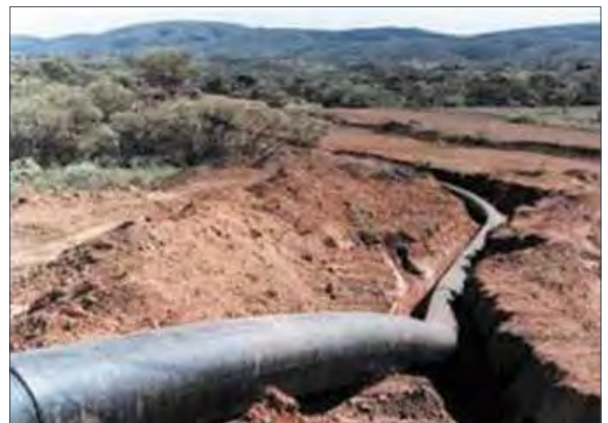
Figure 35b: In-field Laying of Multi-Jointed Pipe
