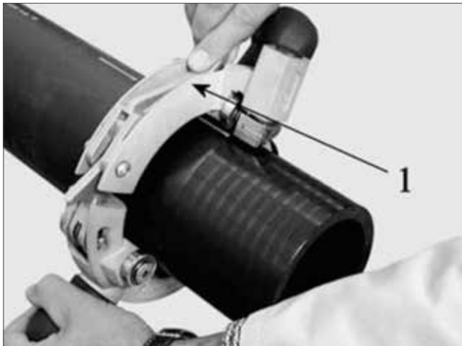
Figure 34: Rotational Peeling Tool Used to Prepare Pipe Ends
